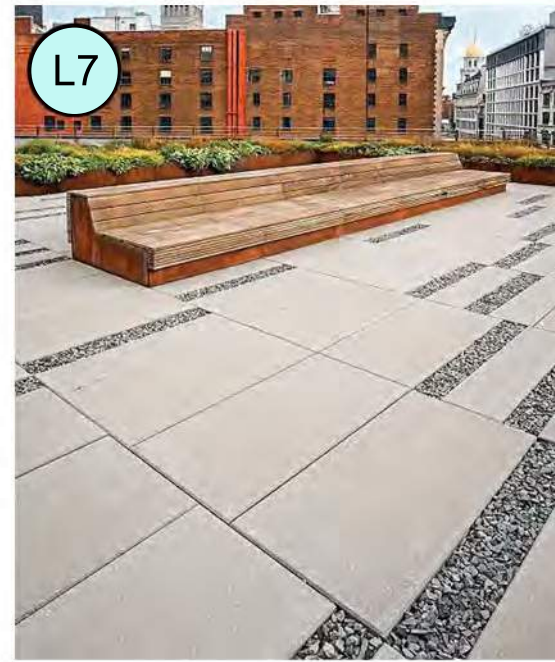
L7 Rooftop Pavers: Hanover Prest
