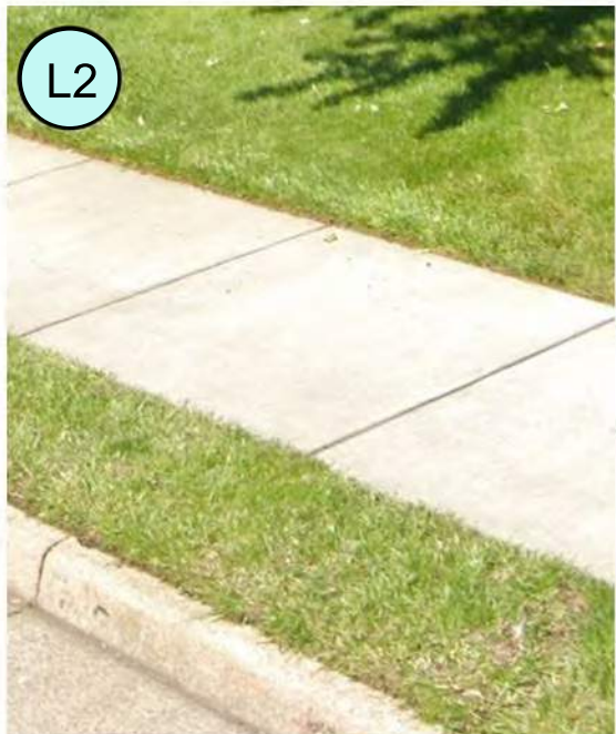
L2 Concrete Paving: Cast in Place
