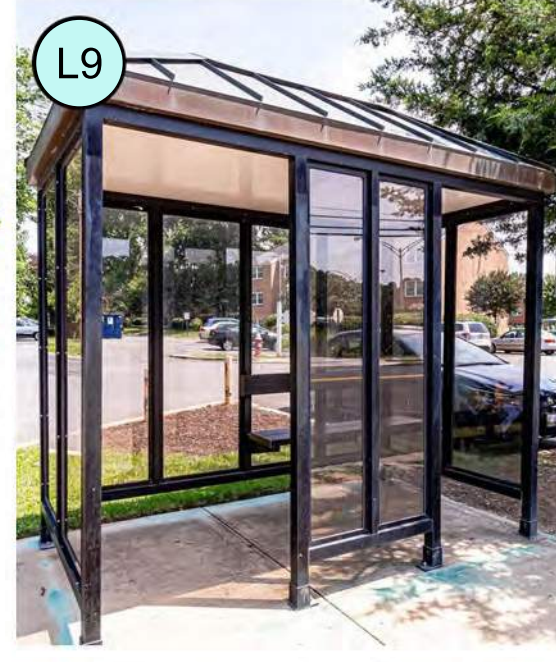
L9 Bus Shelter
