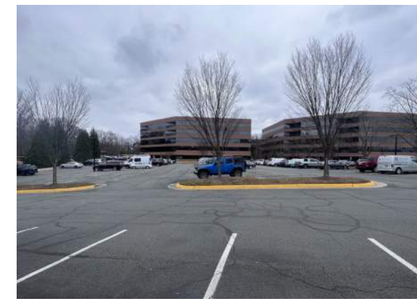
C VIEW LOOKING EAST FROM SITE INTERIOR
