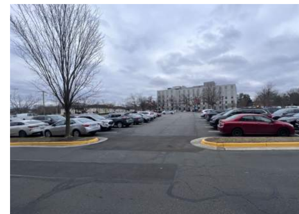
H VIEW LOOKING WEST FROM ADJACENT OFFICE BUILDING
