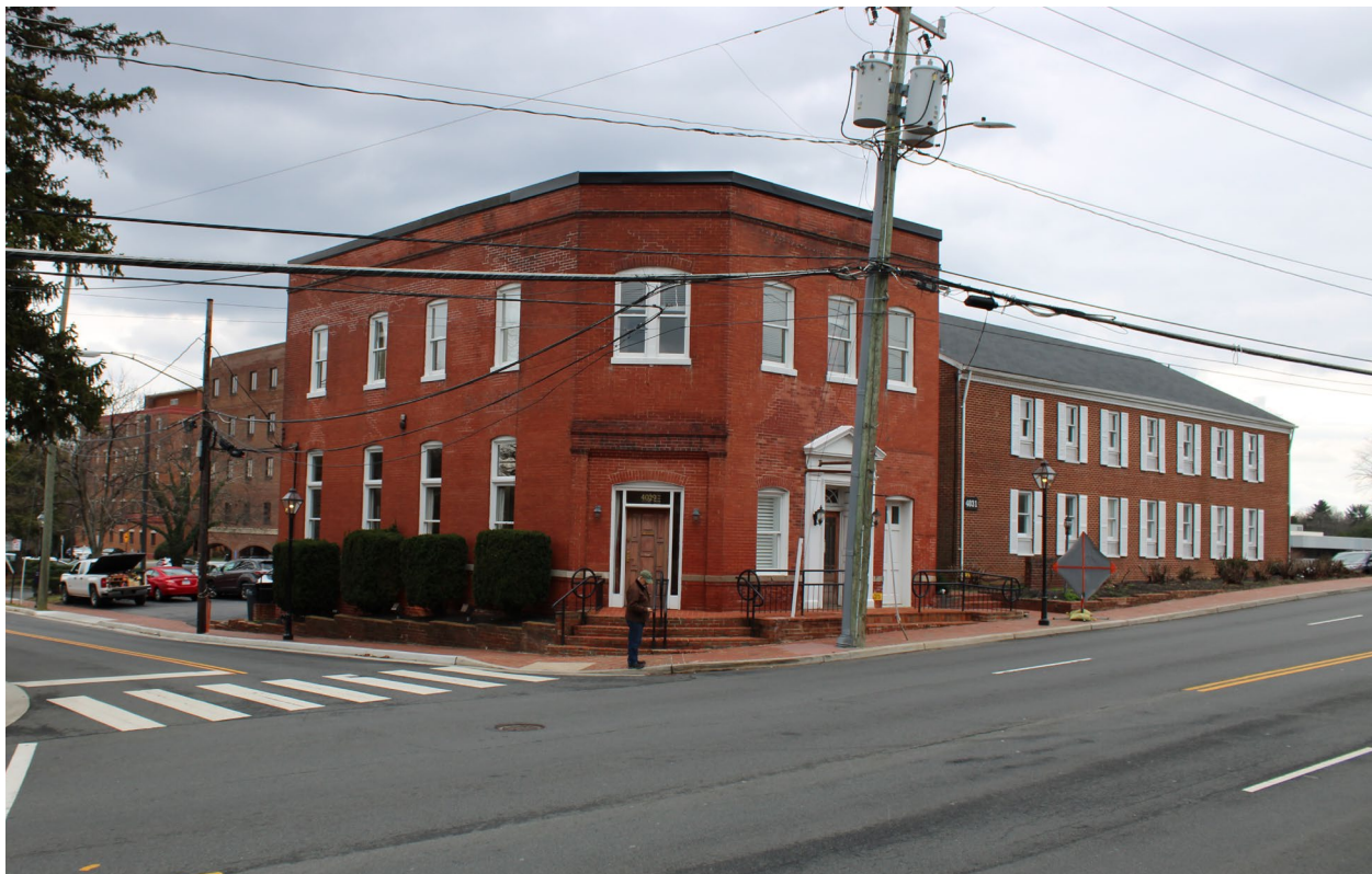
Figure 2: 4029 Chain Bridge Road, looking southeast. EHT Tracerics.
