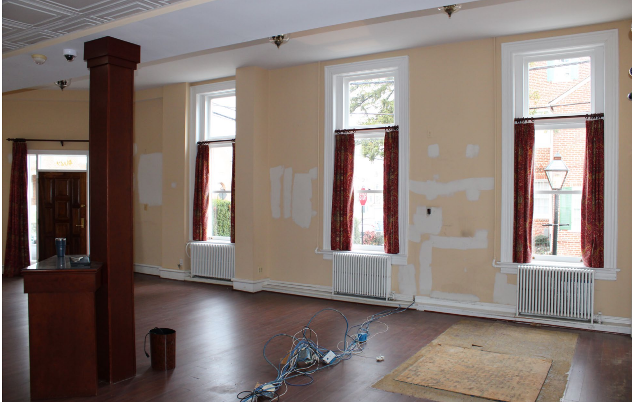
Figure 9: First floor lobby. EHT Tracerics.
