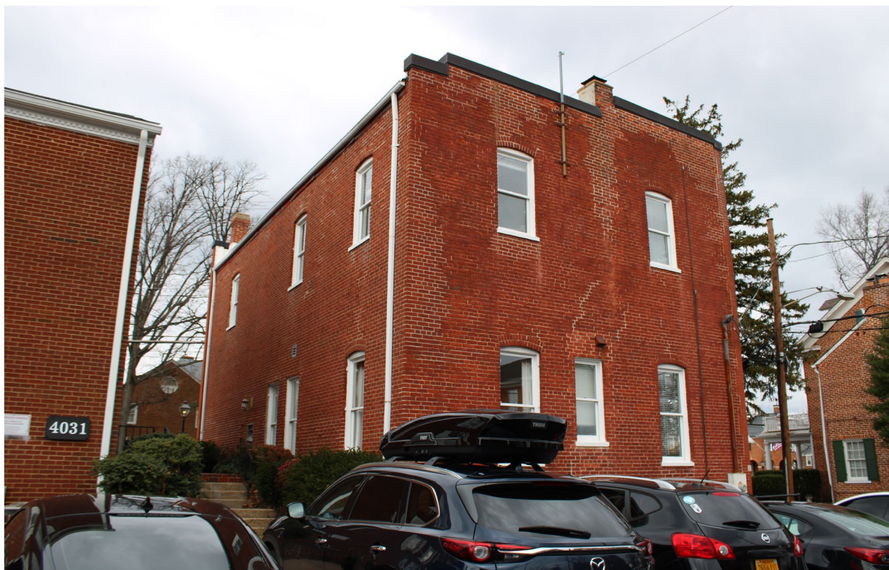
Figure 6: East and south elevation, looking northwest. EHT Tracerics.
