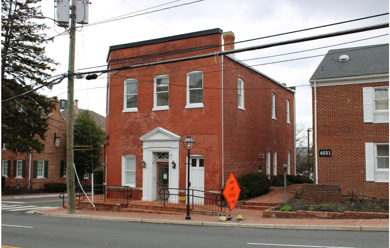
Figure 3: West elevation, looking northeast. EHT Traceries.
