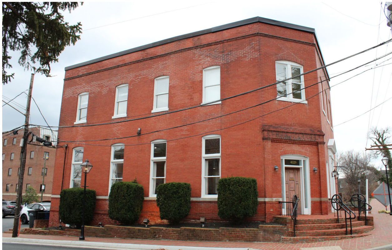
Figure 4: North elevation, looking southeast. EHT Traceries.
