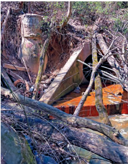
The Mathy Drive culvert experienced severe erosion near two outfalls. The city reinstalled the pipe, added riprap (large rocks) for erosion control and outfall protection, added a headwall to stabilize the pipe and prevent future dislodging, and backfilled the area with fresh compactable dirt.
