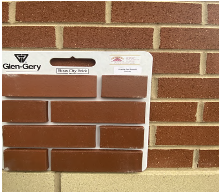
GLEN GERY GRANITE RED VELOUR (PROPOSED) V. GLEN GERY RED CLIFF (EXISTING CENTER)
