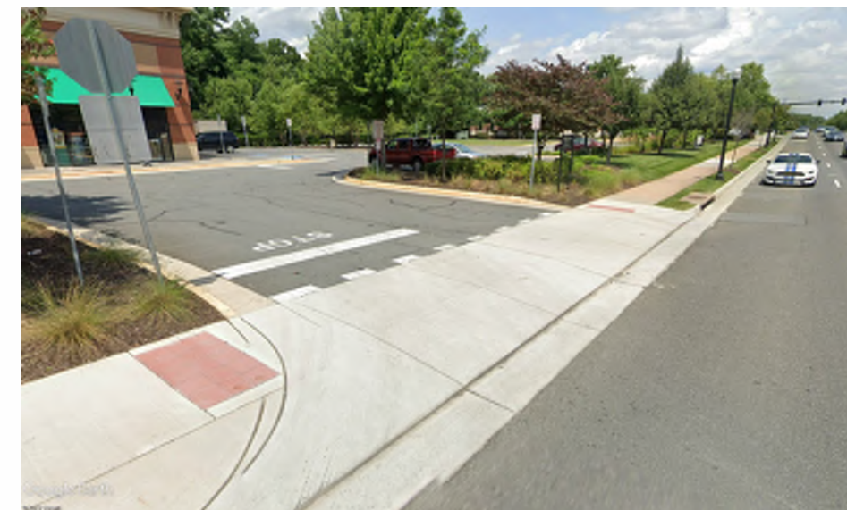
3 Fairfax Blvd: Existing West Entrance
