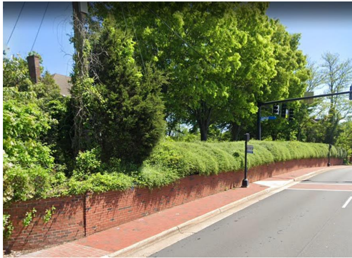
View Along Chain Bridge Road
