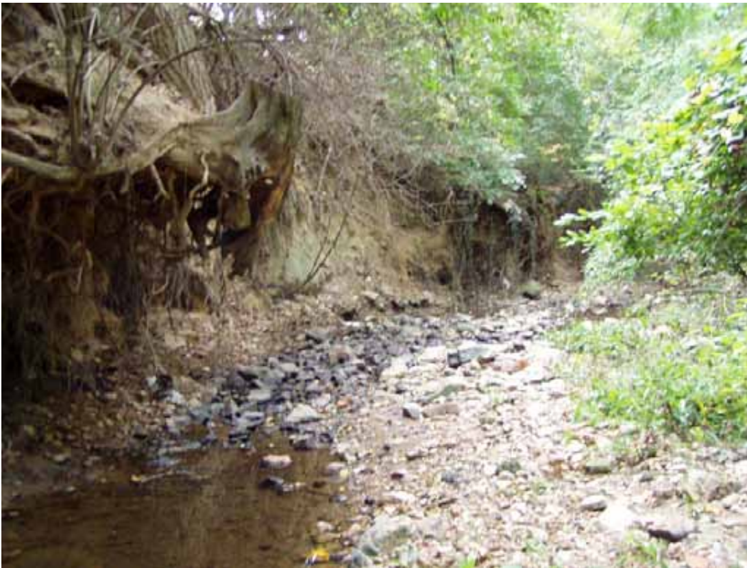
Figure 1-2: Stream Bank Erosion in Accotink Creek near City Historic District
