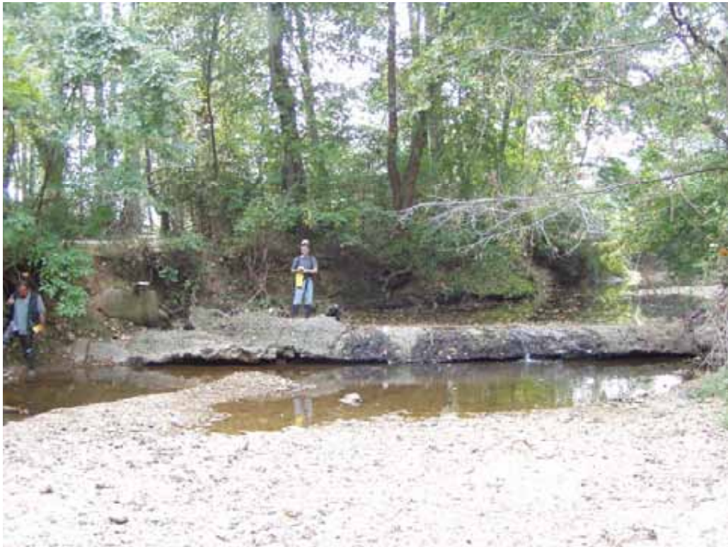
Figure 2-14: Barrier to Fish Movement on Accotink Creek Downstream of Daniels Run
