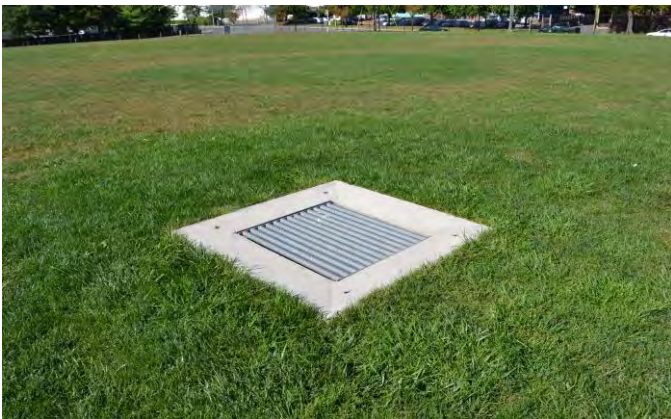
Drain in center of field
