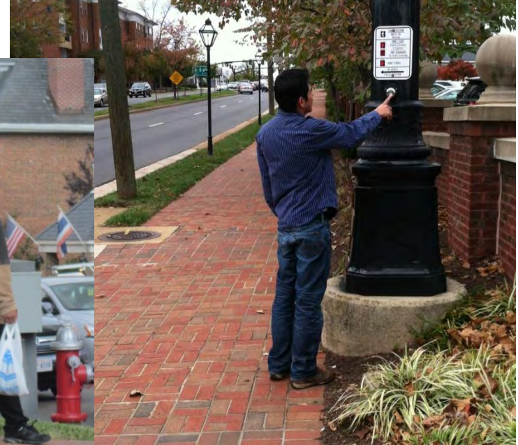
Non-ADA accessible pedestrian signal pushbuttons
