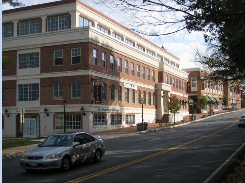
Chain Bridge Road North
