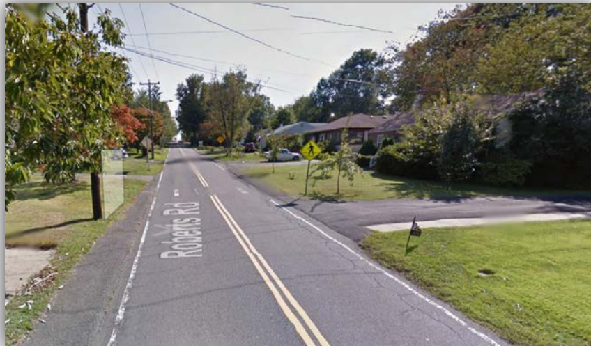
Existing Condition at South End
