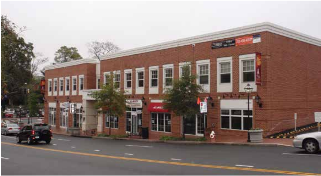
After utility lines were placed underground
