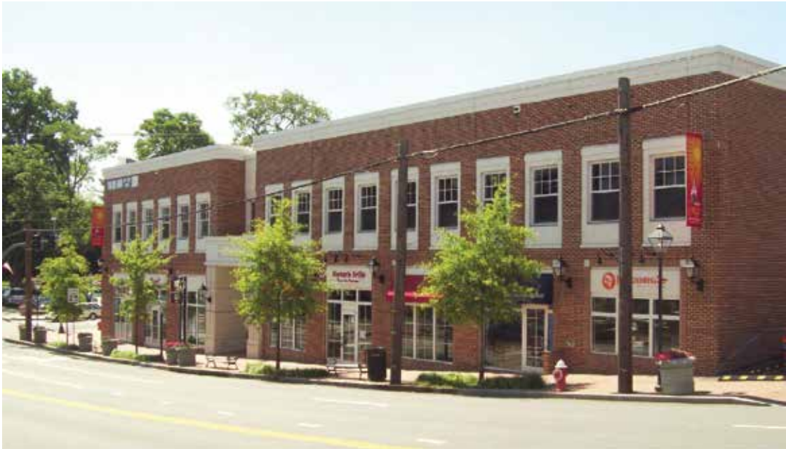
Before utility lines were placed underground
