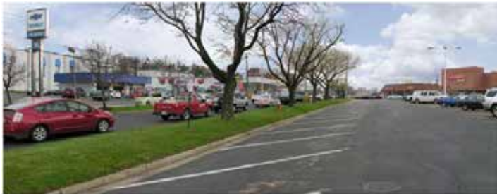
Fairfax Boulevard today is a highway built primarily for cars.
