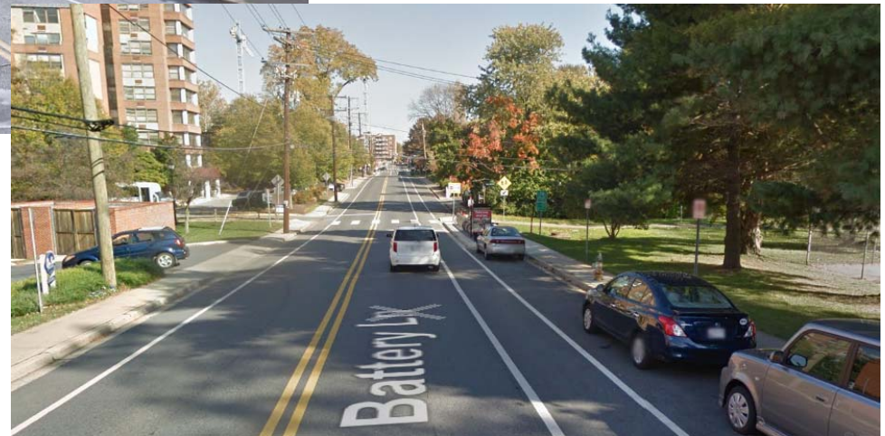
Battery Lane in 2014 with two-lane section, bicycle lanes, and parking on south side
