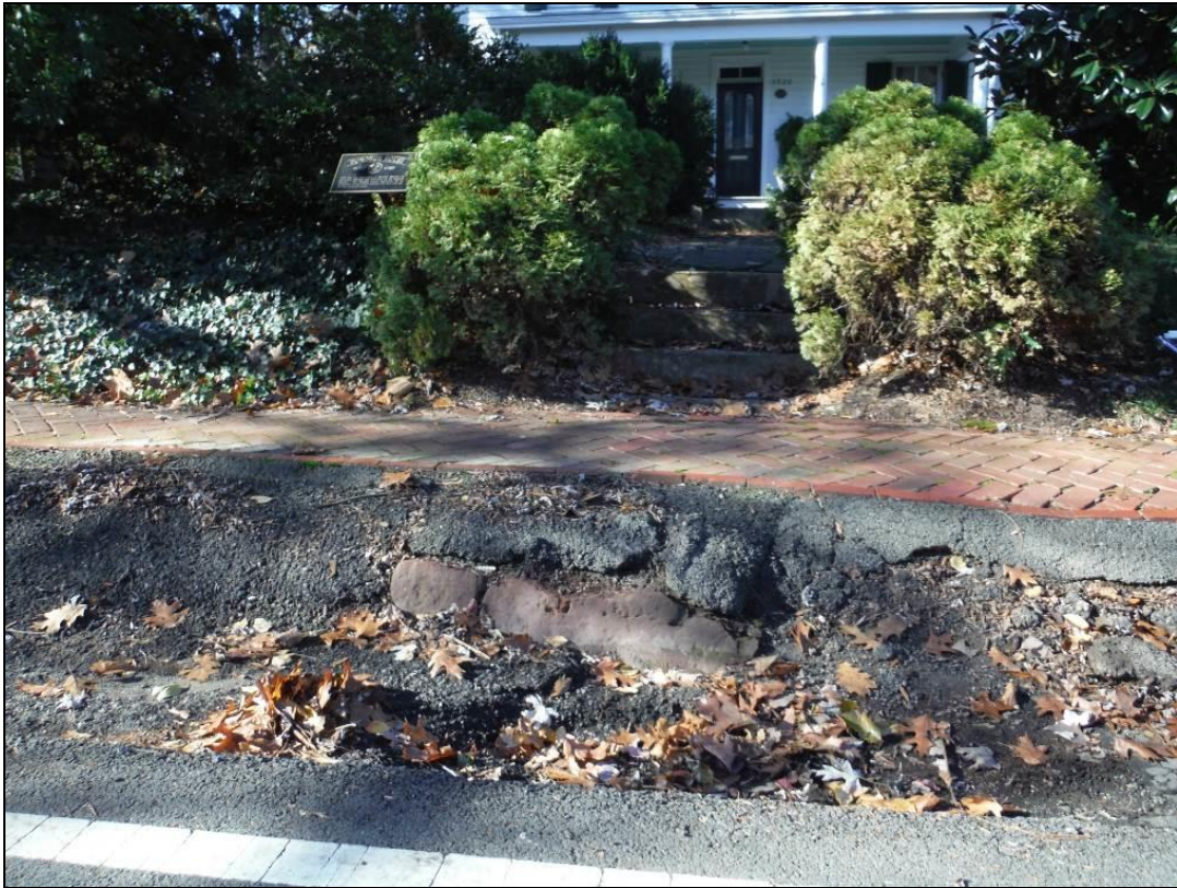
Photo 13: Original Step/Stoop Under Modern Sidewalk at 3920 Chain Bridge Road, Facing West.
