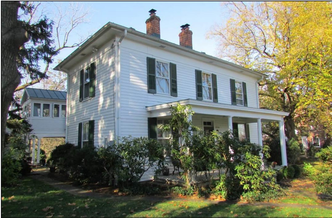
Photo 3: The House at 3920 Chain Bridge Road (151-0003-0019), Looking Northwest.
