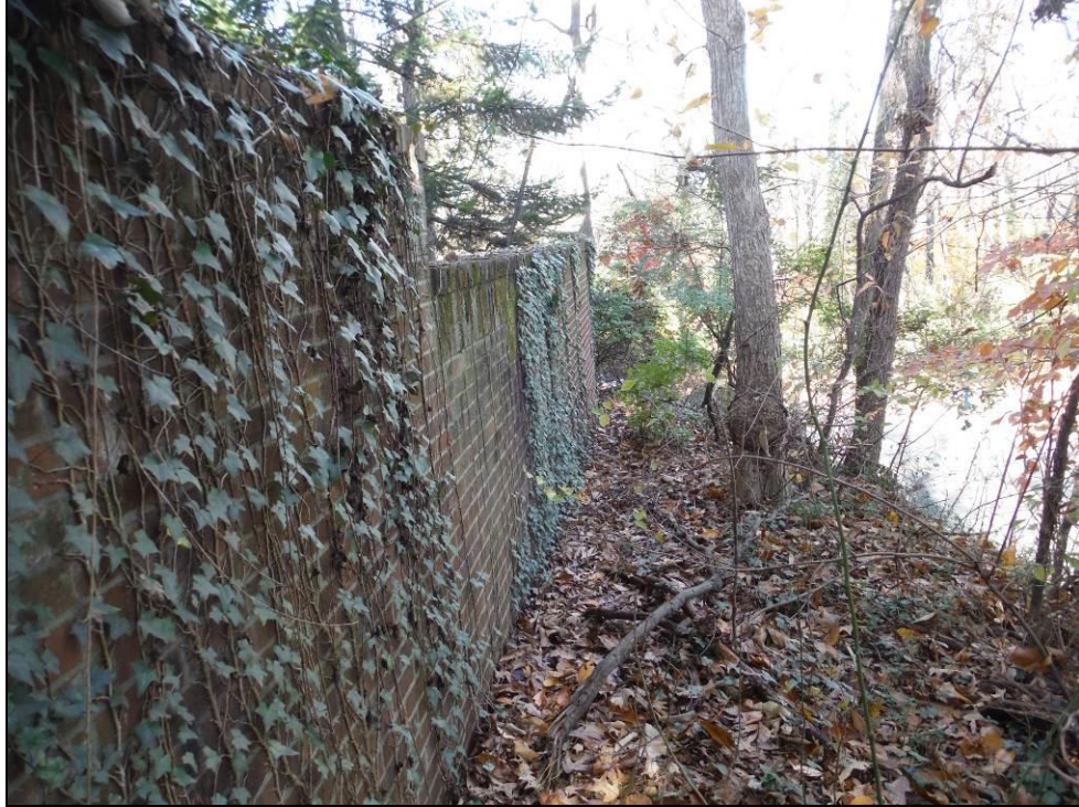
Photo 9: Facing North from Near STP A-16.
