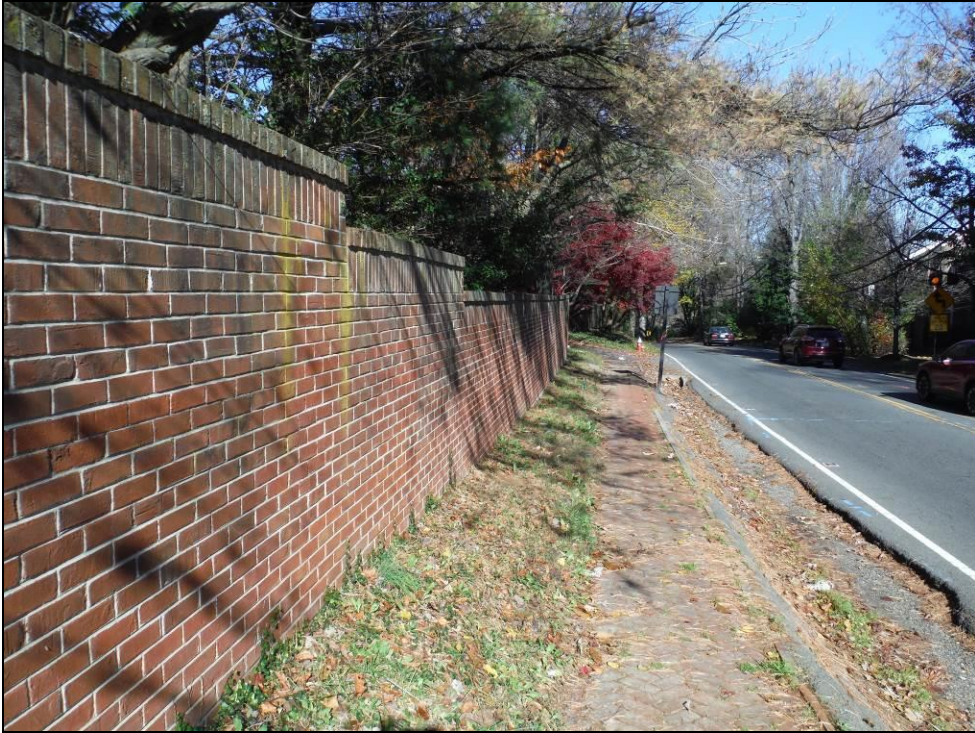
Photo 7: Facing North Along Existing Sidewalk from Near STP A-9.
