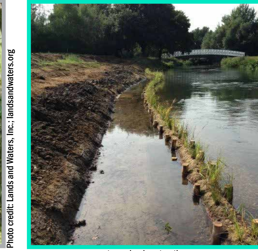
stream bank restoration
