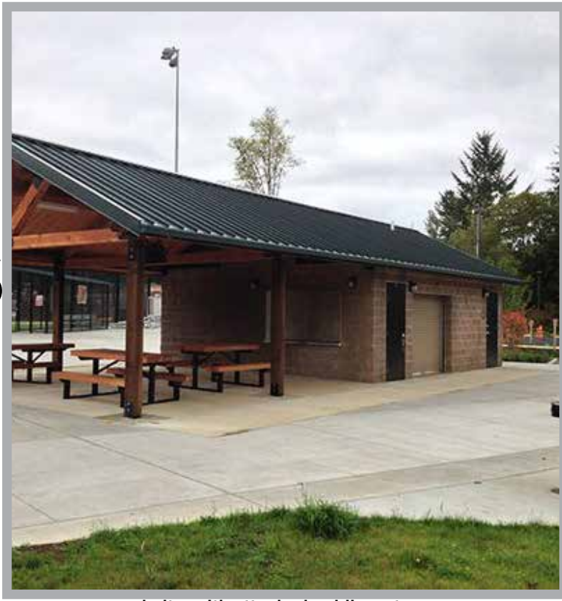
shelter with attached public restroom
