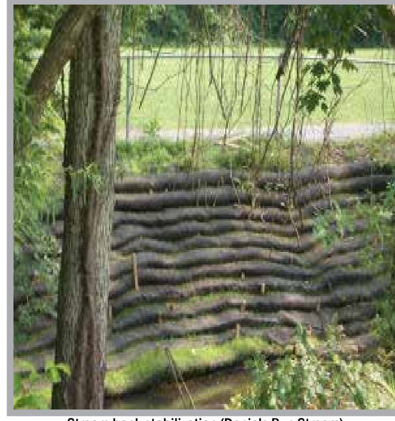
Stream bank stabilization (Daniels Run Stream)
