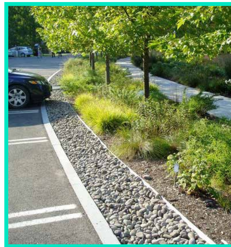
infiltration median with shade trees and shrubs
